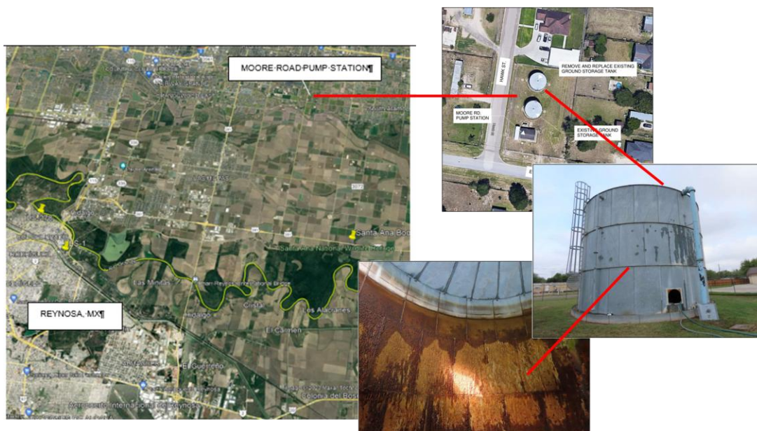
Figure 3 MOORE RD BOOSTER STATION
